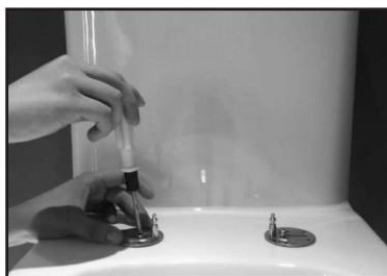
2. Tighten the screws but not to the end in order to adjust the seat cover properly
