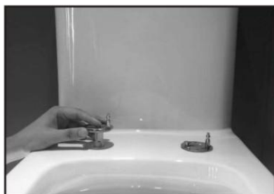
1. Insert the fitting including plug and screw into the hole on the toilet
